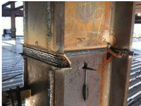
Figure 1.1.3. Post-Northridge welded column splice
